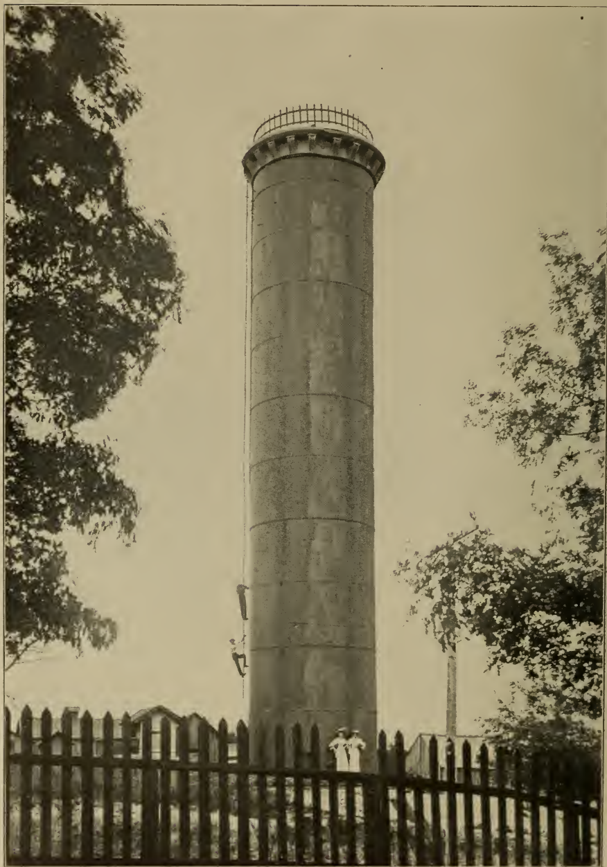
STAND PIPE—ROCK ISLAND, ILLINOIS.
